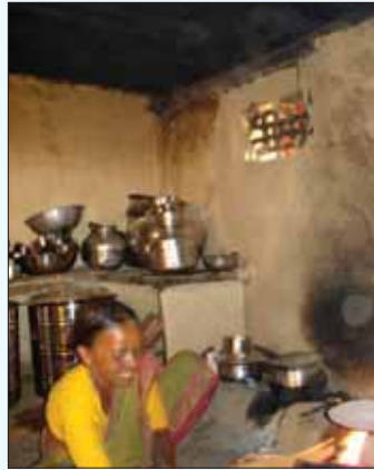
The effects of cooking over an open wood fire indoors. Note the ventilation 'window,' and the condition of the smoke blackened walls and AC ceiling. The occupants have lived in this dwelling for 16 years.
