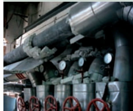
Broken and exposed asbestos piping
