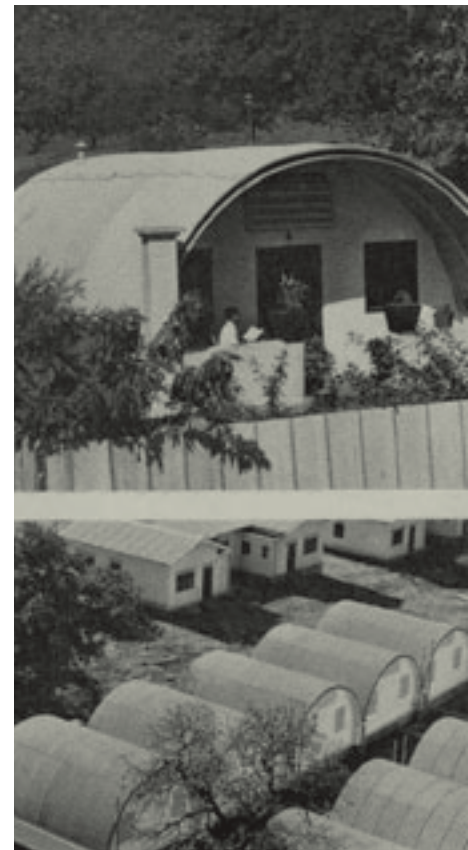
Asbestos cement housing in India
