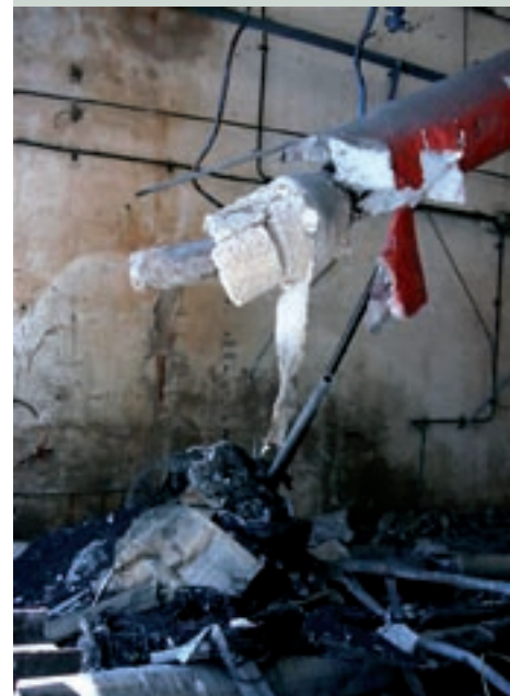
Broken and exposed asbestos piping
