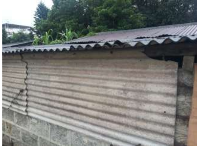
Asbestos sheet were used as roof
