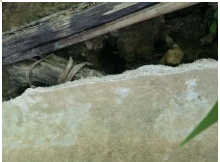
asbestos are serious damaged
