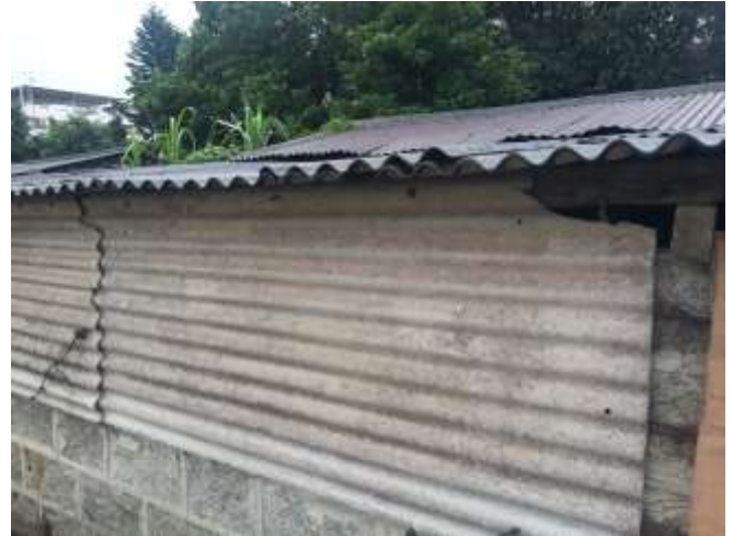
Asbestos sheet were used as roof
