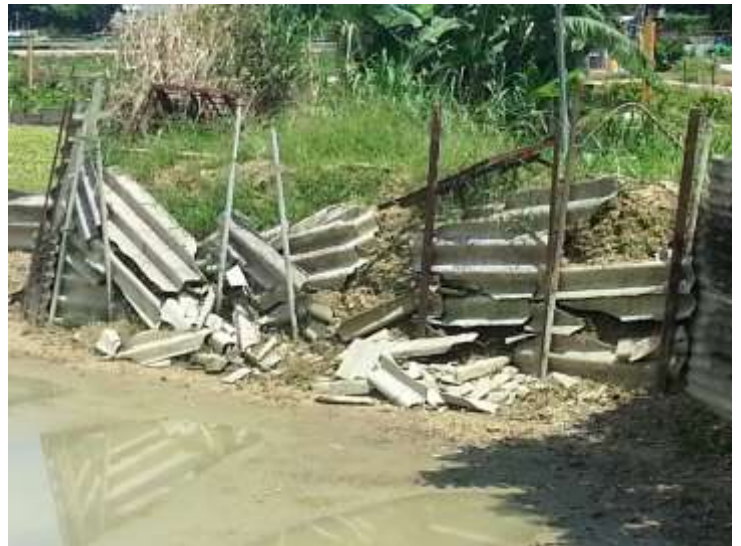
asbestos are serious damaged
