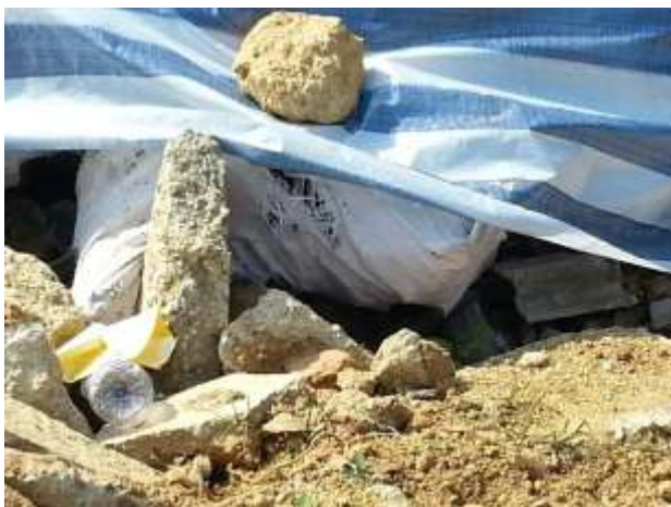
Broken asbestos was just covered by canvas
